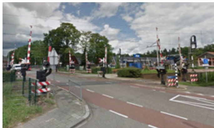
Spoorwegovergang Den Dolder
